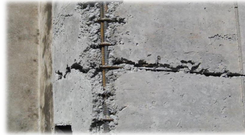
Problems with congested reinforcement
