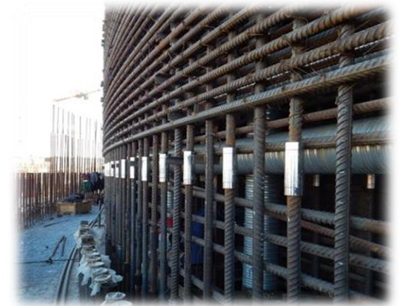
Construction of Belarusian NPP II
