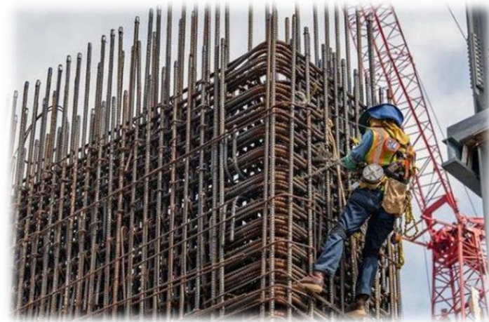
Problems with congested reinforcement
